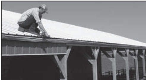
Josh works to fix the gutter in the Hoover herd bull run.
